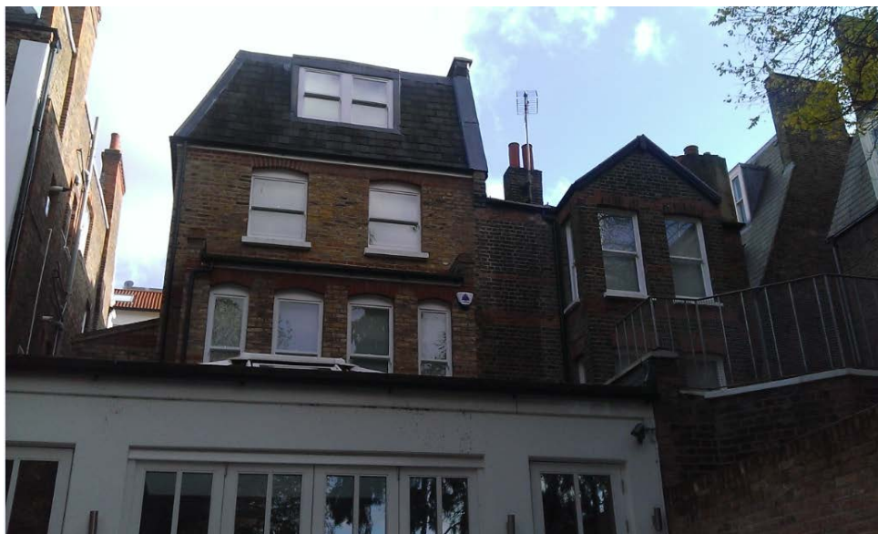
Rear elevation comprising ground, first, second and mansard levels.
