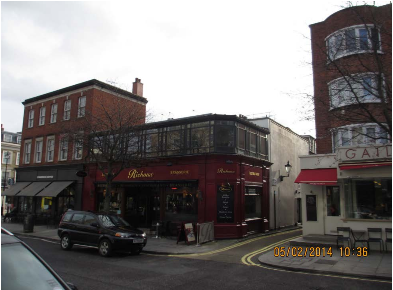
Application site as seen from Circus Road.
